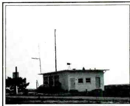
The transmitter building at the East Moriches, New York Coast Guard station.
