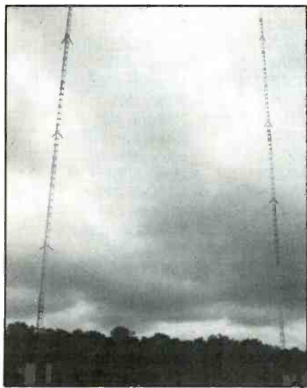
WLIM's two transmitting towers. Lens distortion makes it look as if they're not quite vertical. At one time there was a third tower but that one was razed several years ago. (Photo by Tony Earl)
